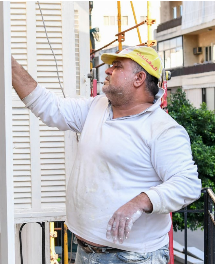
Rehabilitation works in Beirut December 20, 2020
