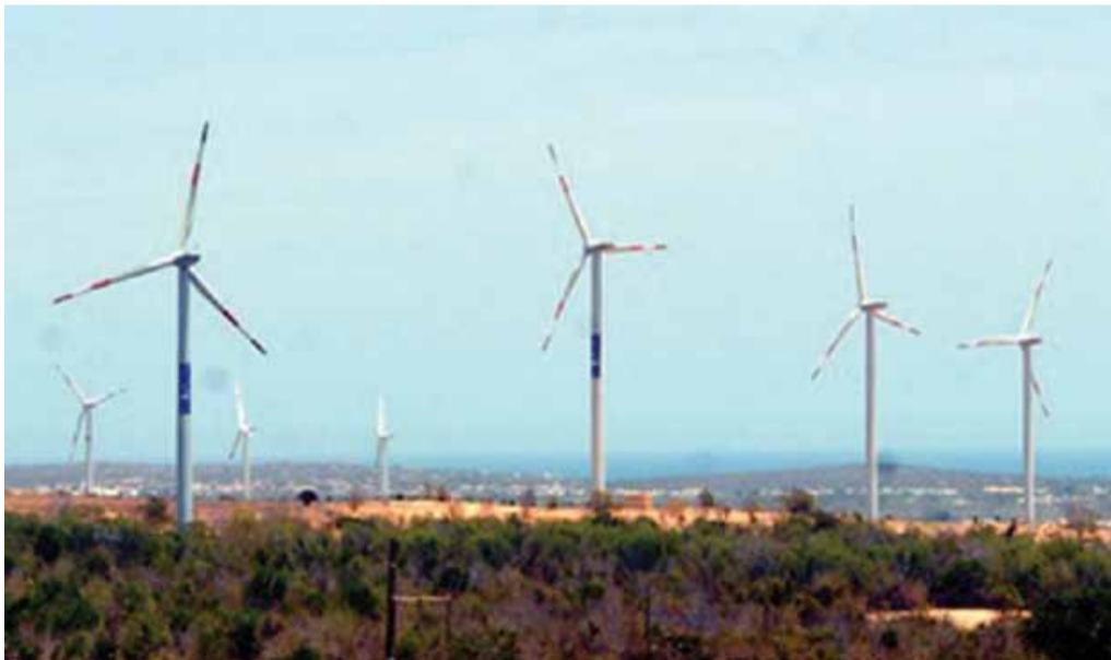
Wind turbines at the Tuy Phong Wind Power Plant in Binh Thuan province.
